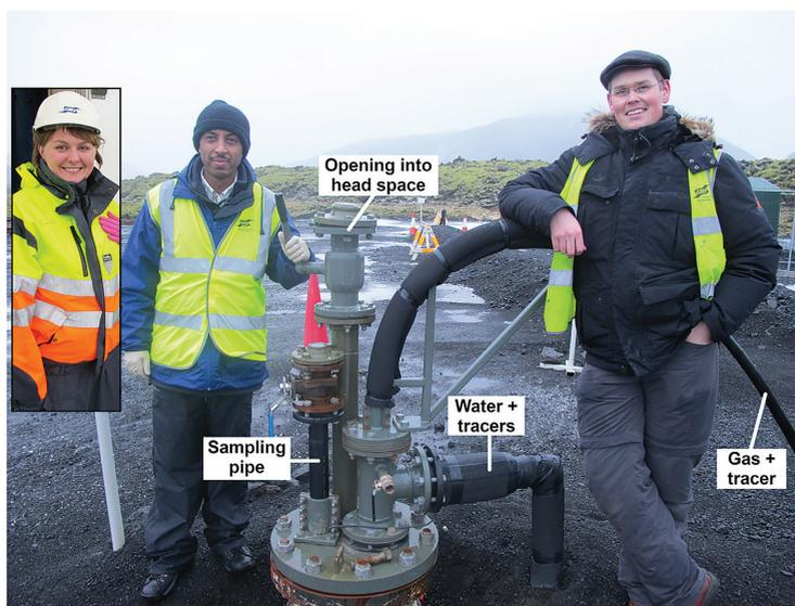
**Figure 4.19** The HN-02 injection wellhead with the attached polybutylene CO<sub>2</sub> gas pipe, polyethylene water pipe, sampling pipe for high pressure sampler and video camera, and opening into the headspace above the water level. The graduate students that monitored the well fluids before, during and after the injection are also shown from left to right; Sandra Snaebjornsdottir, Kiflom Mesfin, and Helgi Alfredsson.
